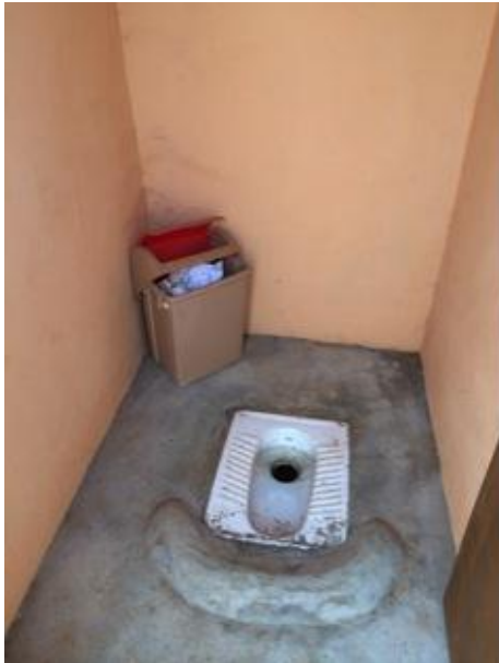
FIGURE 4-7 TAHA POUR-FLUSH INTERIOR
