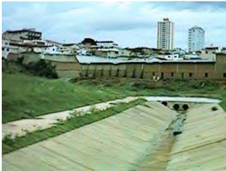
Figure B-2: Storm water channel, image taken at the source of the Jardim de Boa Esperança stream
