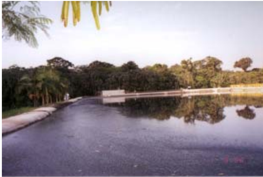
Figure 13: Anaerobic Lagoon
