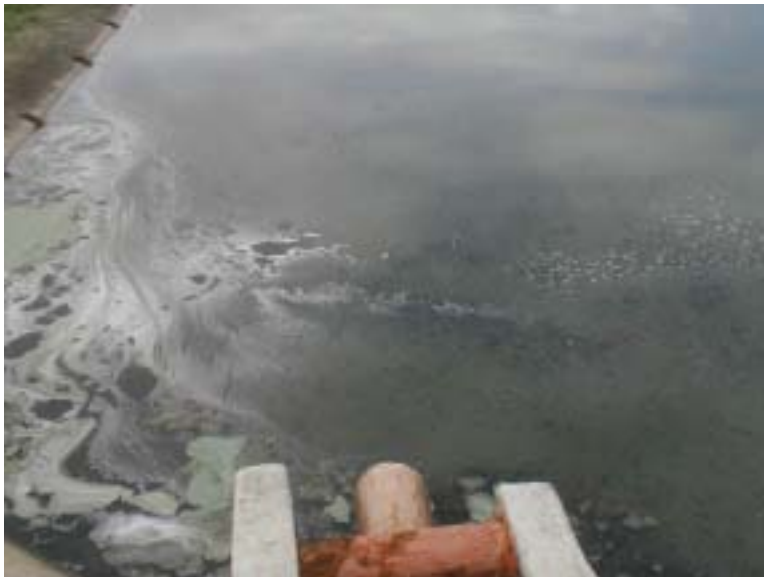
Figure 28: Floating ‘Sludge Bombs’ in the Facultative Lagoons
