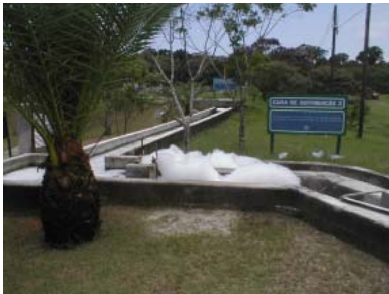
Figure 29: Formation of Foam at the Exit of the Anaerobic Lagoon
