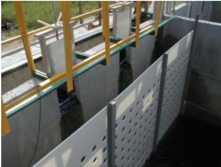
Figure 10: Entrance to the CEPT Clarifier Tanks
