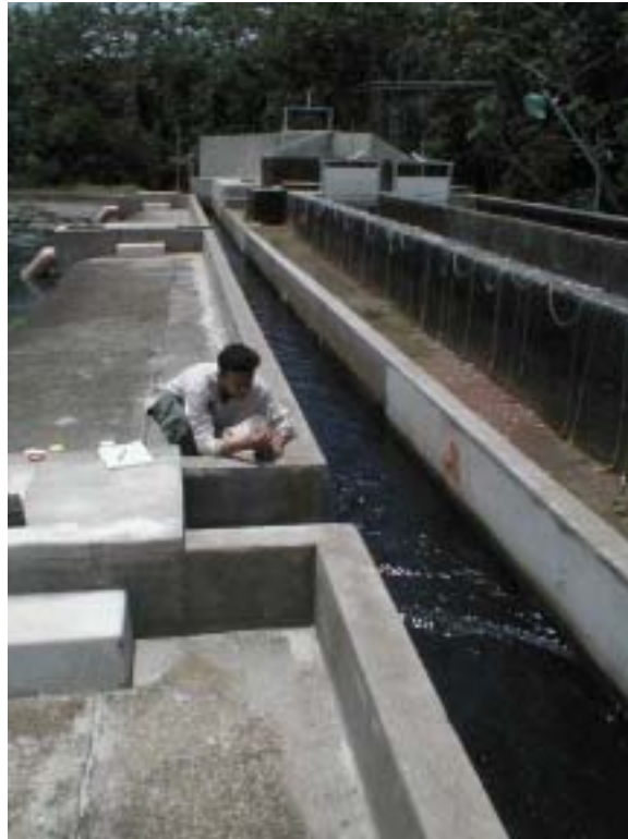
Figure 23: Sampling Point I-3, Inlet to the Anaerobic Lagoon
