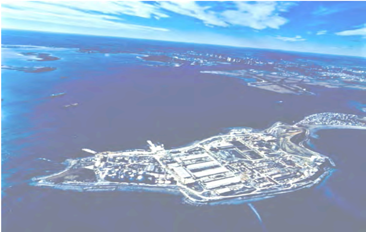
Figure 5-1: Boston Deer Island Wastewater treatment plant ( http://www.bryant-engrs.com/projects/deer.htm )
