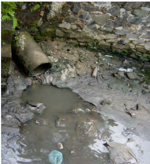
Figures 1.5: Sewage Discharge into stream
