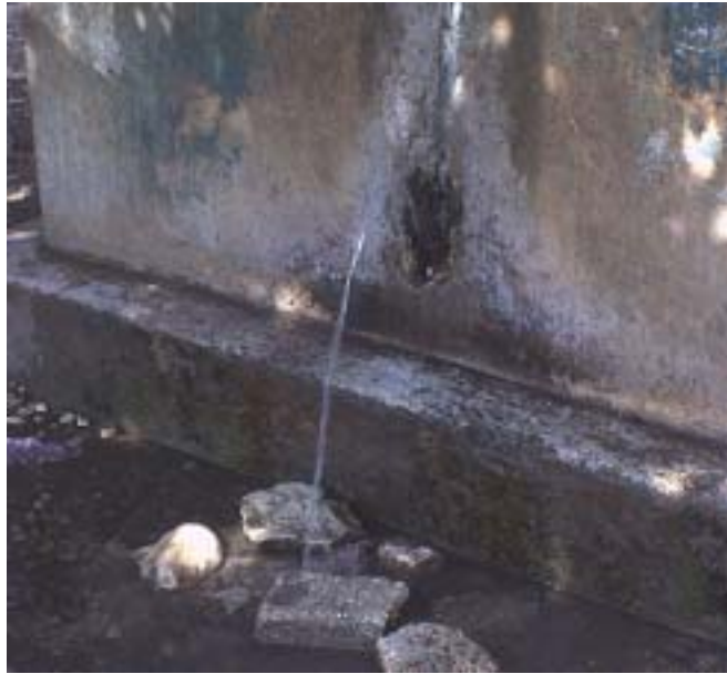
Figure 6-3. On-Site water source for 01/13/01
