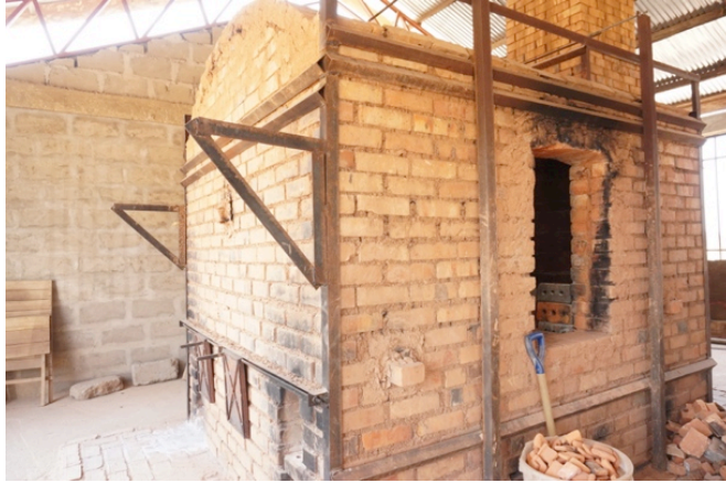
Figure 3-8 The kiln in PHW
