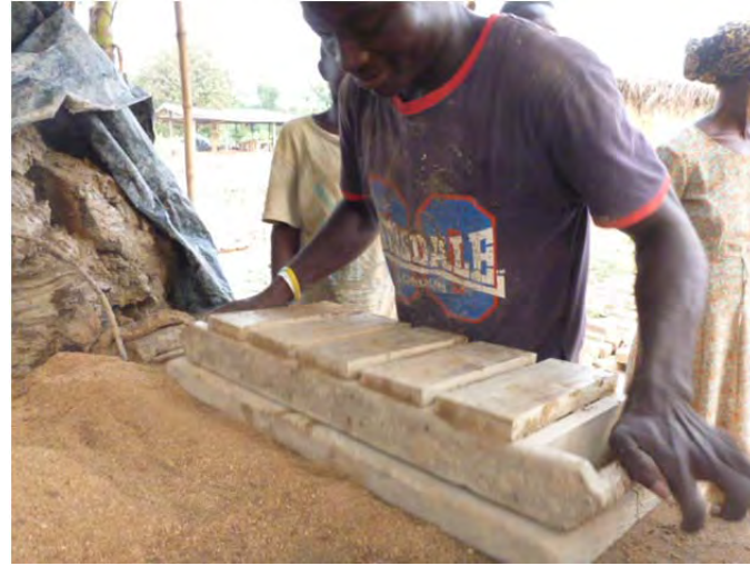
FIGURE 11 - HAND MOULDING GREEN BRICKS
