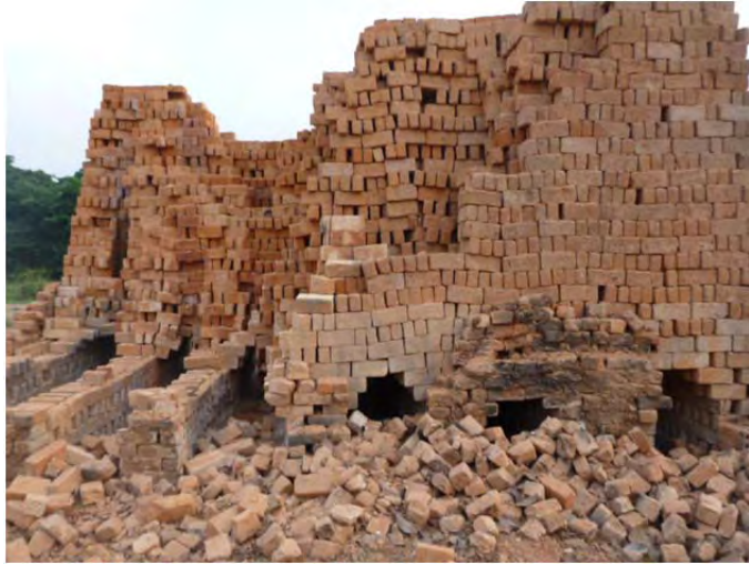
FIGURE 10 - PARTIALLY DECONSTRUCTED CLAMP KILN
